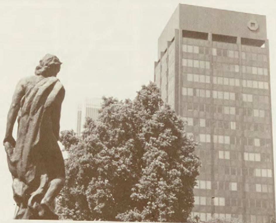
Chase Bank AG in Frankfurt am Main
